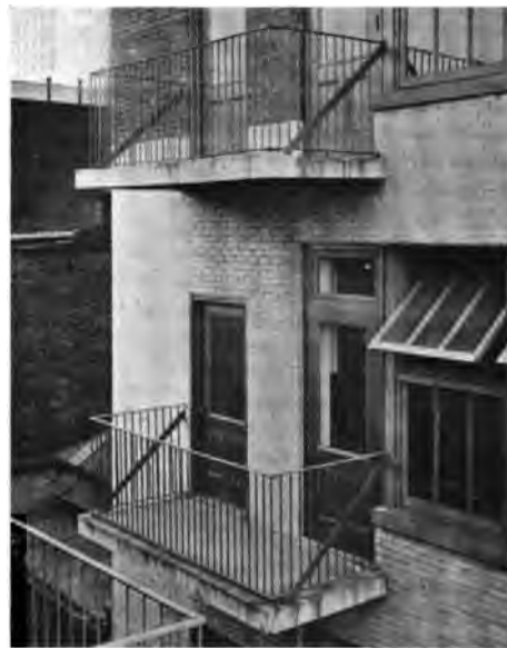
Fig. 4. Smoke-Proof Tower with Balcony Entrances.*
